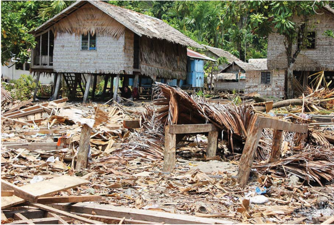
Figure 3– Damage in Venga Village, Nendö Island [Photo: Matt Anderson/DFAT/AusAID]
