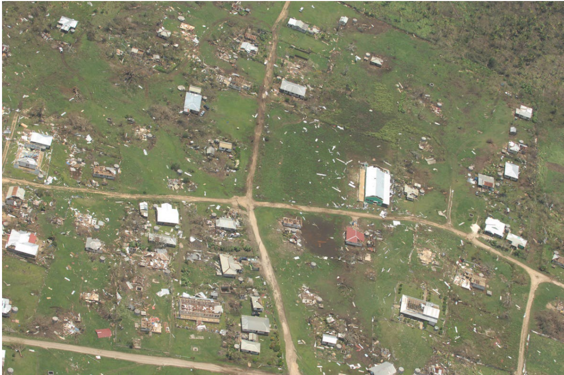
Figure 4– Damage to homes on Lifuka Island, Ha’apai, Tonga [Photo: New Zealand Air Force]
