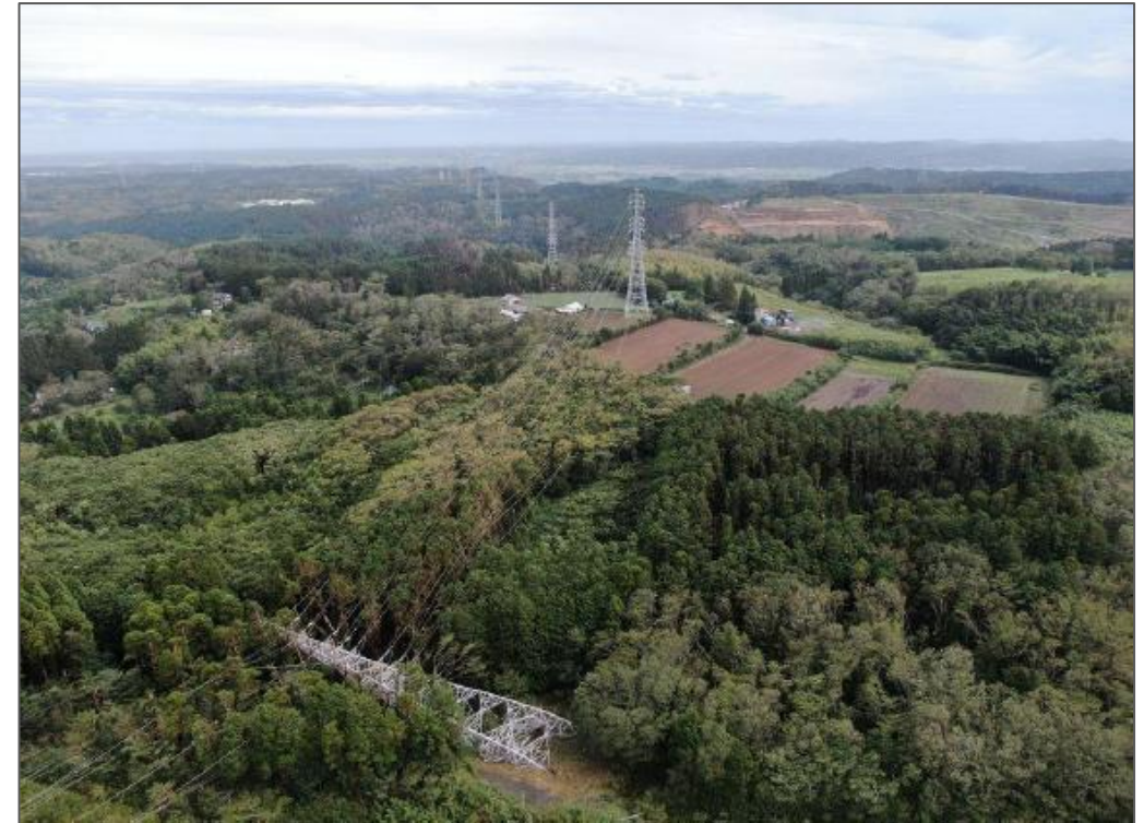
(TEPCO Power Grid)
